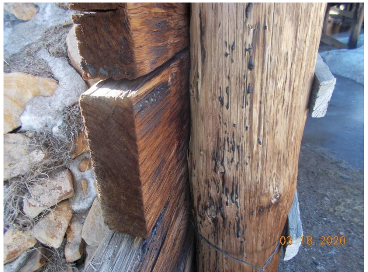
Suspect asbestos-containing material I-13-H-TR02. The tar material is non-detect for asbestos.
