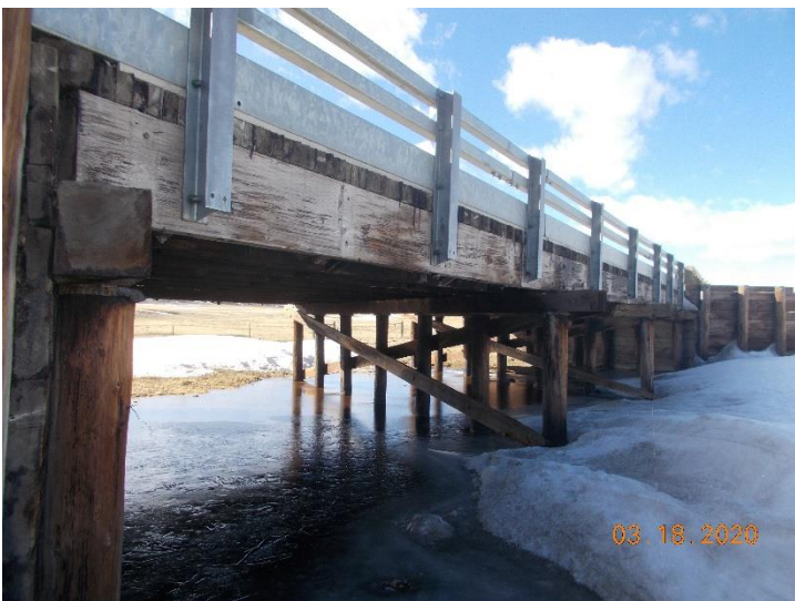
View beneath bridge looking southwest.
