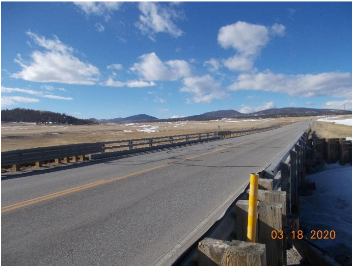
View of bridge I-13-H looking southwest.
